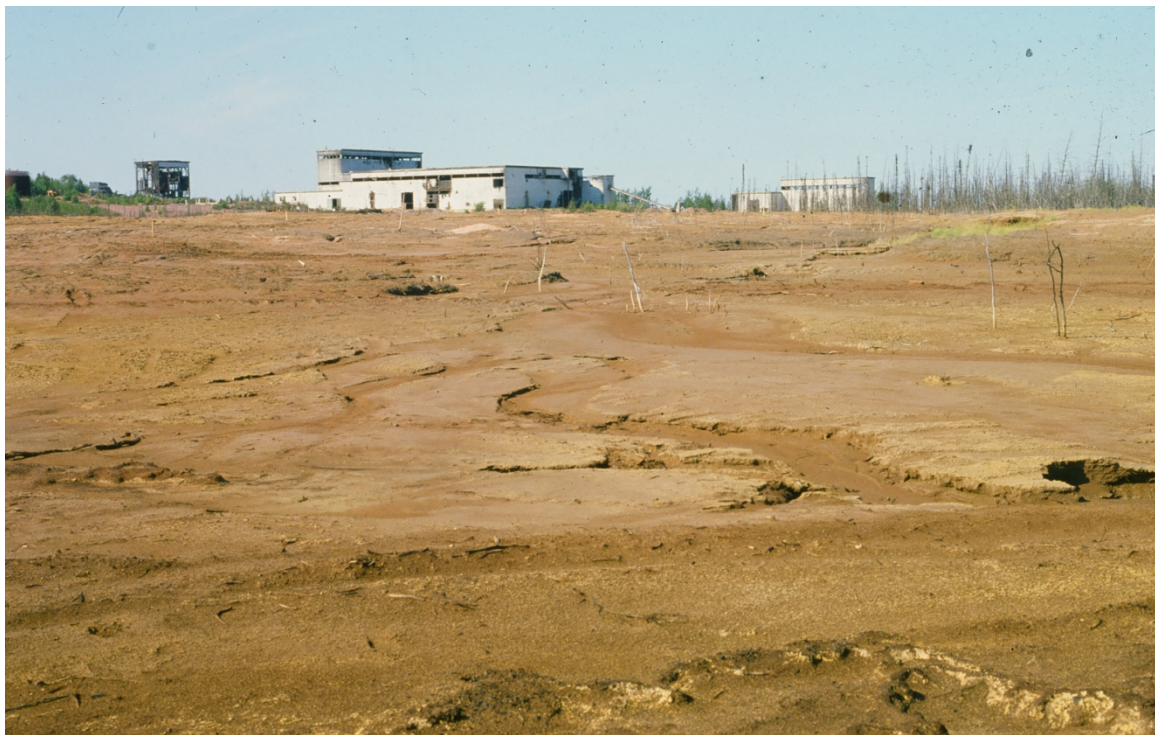
Photo 2: Lorado mill and tailings looking west (circa 1978 - prior to mill dismantling)
