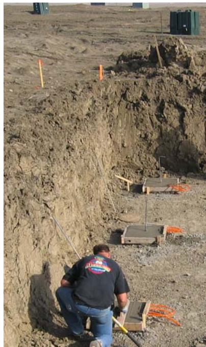
Figure 3: Leveling of the piling caps
