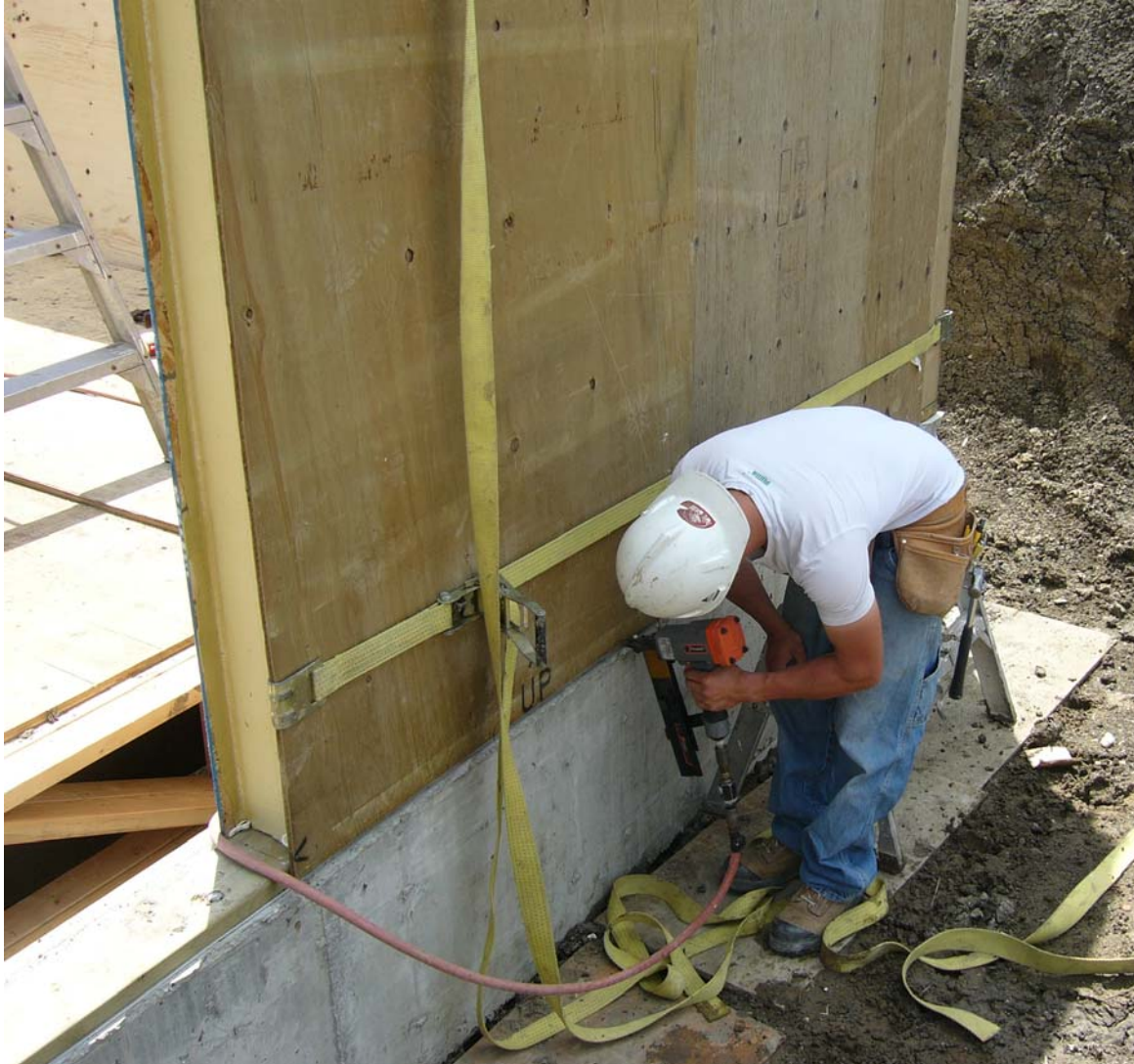
Figure 5: Concrete grade beam and the SIPs for the basement walls
