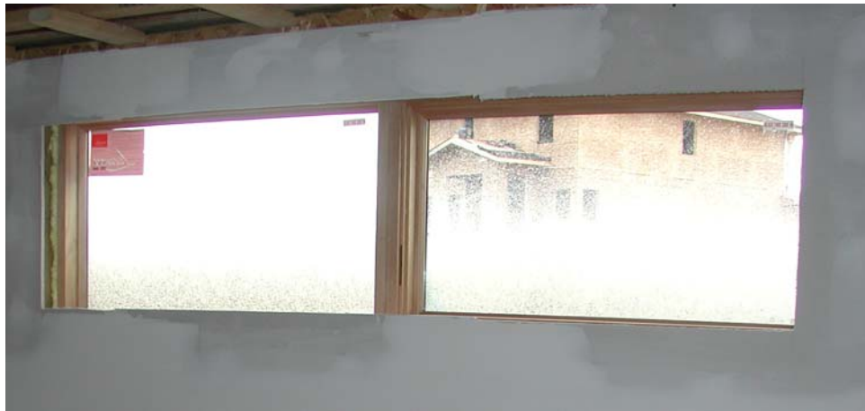
Figure 13: South facing windows in the basement of the house
