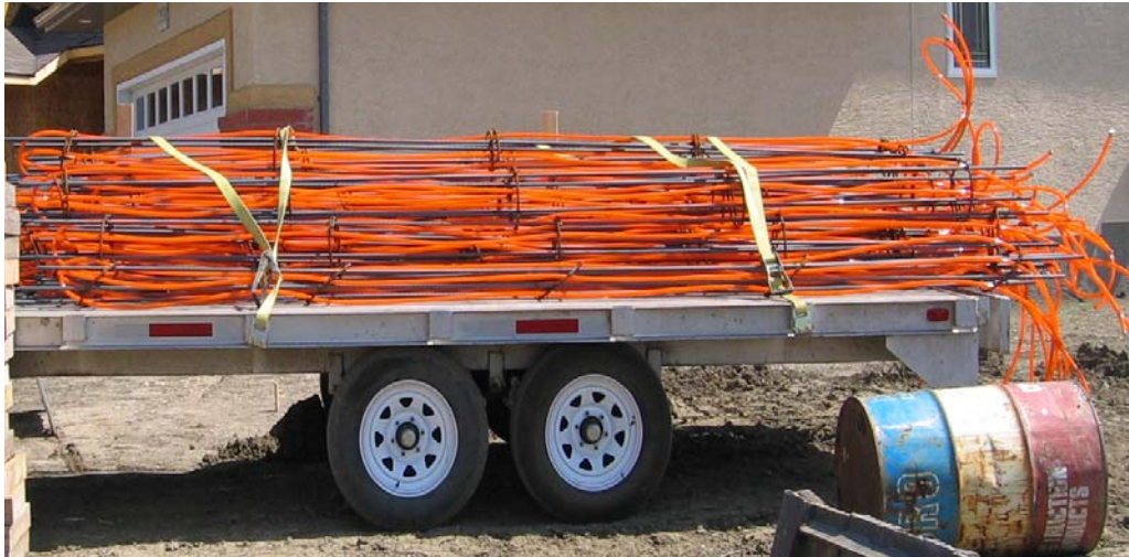
Figure 2: Rebar and plastic cooling pipes for the pilings
