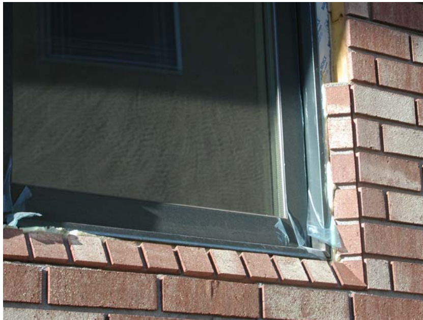
Figure 12: Window installed in an east-facing wall
