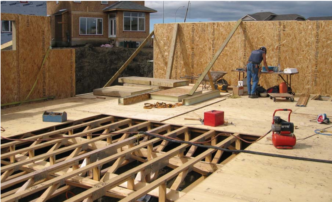
Figure 4: Basement floor with wood trusses
