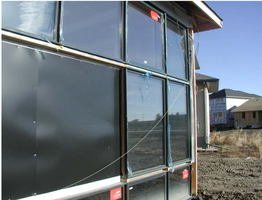
Figure 15: Active solar heating panels being installed
