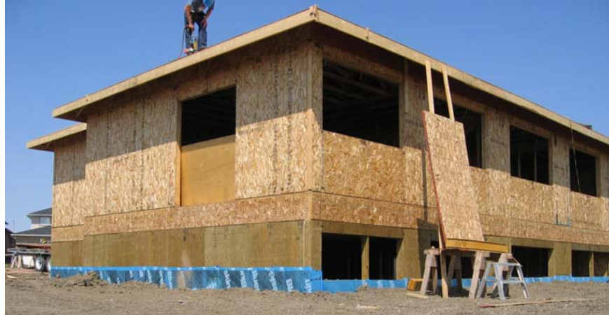
Figure 9: View from the southwest as framing is nearing completion
