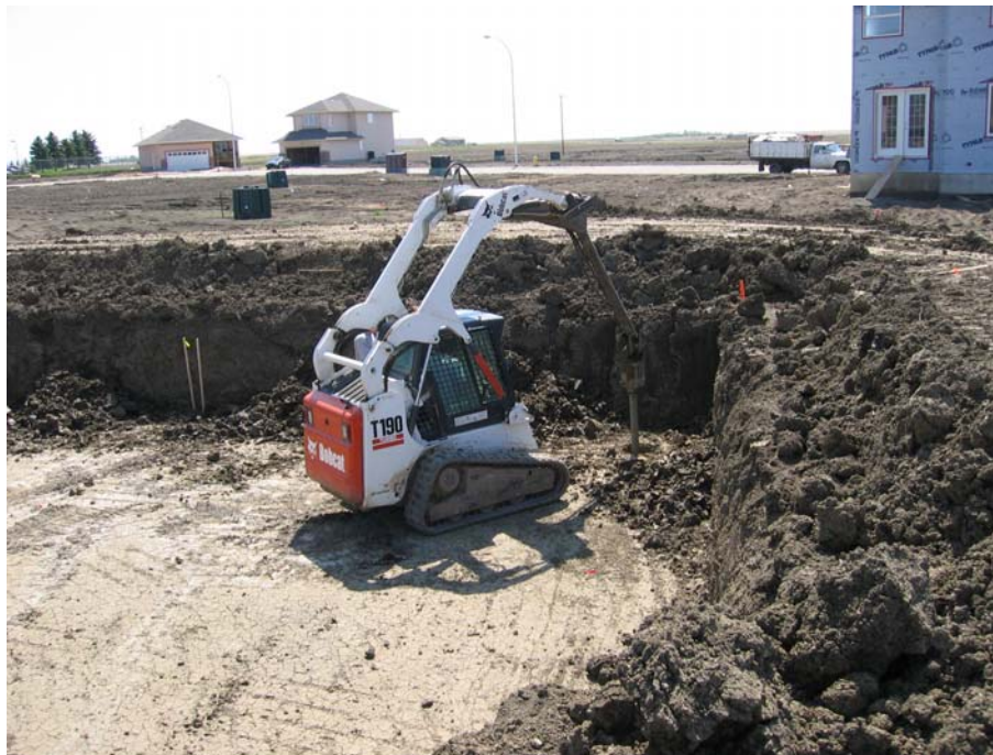
Figure 1: Basement excavation and drilling of the piles for the home
