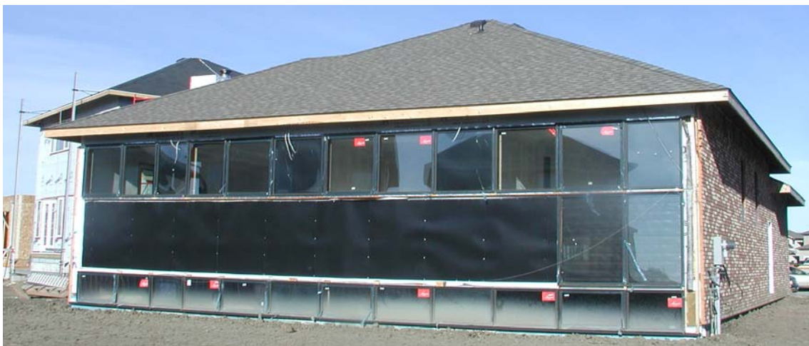
Figure 14: View of the south side of the house
