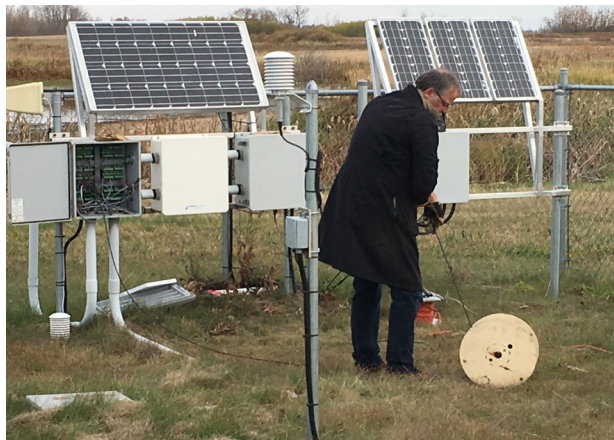
Some re-wiring 11 Oct 2017 Photo: R. Jansen
