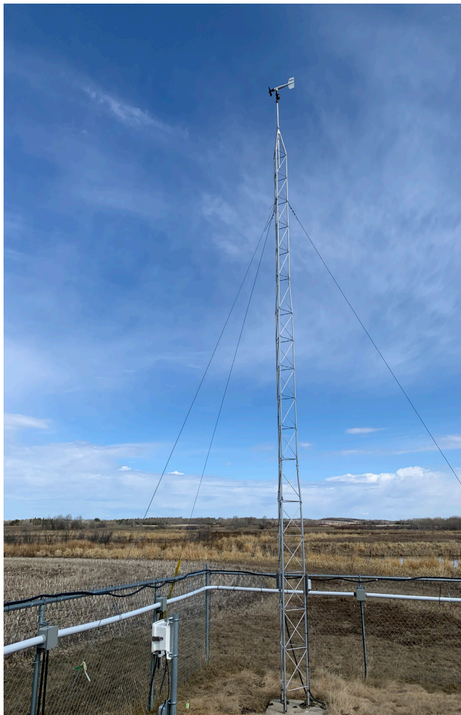
10 meter wind speed and direction tower May 2020 Photo: Development Engineering and Manufacturing
