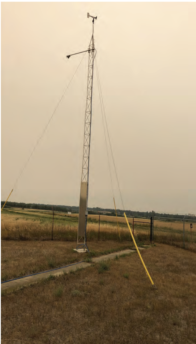
10 Metre Tower with Wind Speed and Direction on a very smoky day 16 August 2021 photo: V. Wittrock
