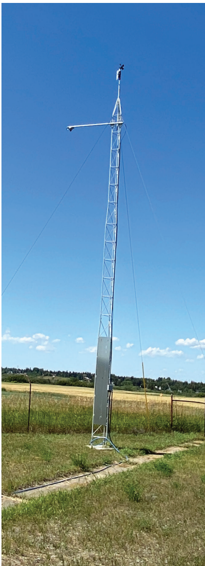
10 meter tower wind speed and direction sensor 08 August 2022 Photo: V. Wittrock
