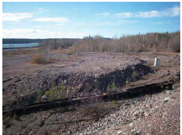
1229 – Debris covered with clean waste rock.
