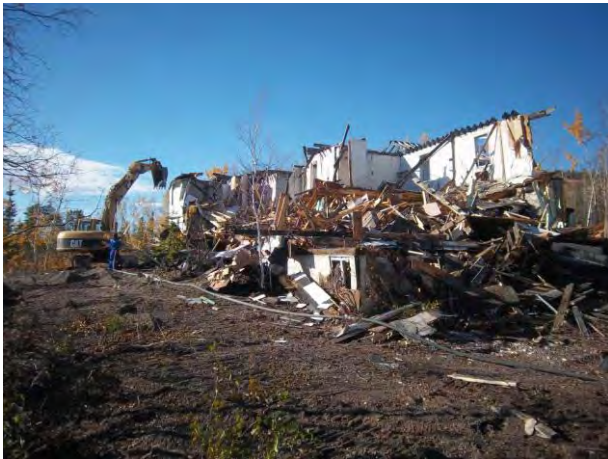
1152 – Demolition of bunk house #4.
