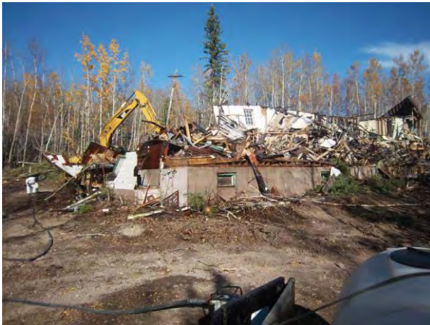
1165 – Demolition of apartment building #4.
