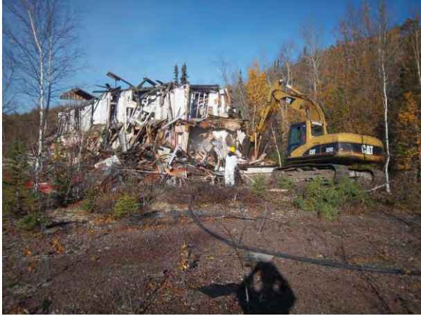
1144 – Demolition of bunk house #1.
