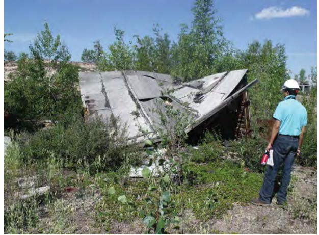
Photograph 30 ↑ Cabins East of Mine-02
