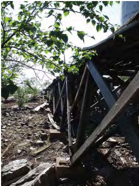
Photograph 111 ↑ Tailings and Utilidors-01
