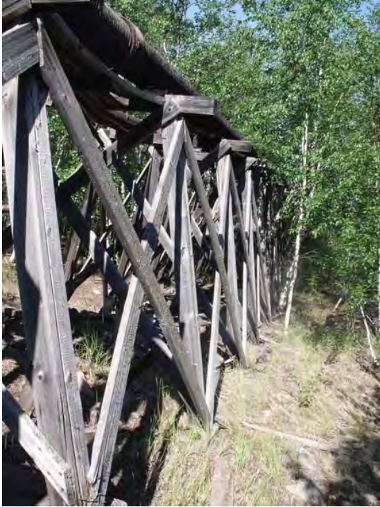
Photograph 113 ↑ Tailings and Utilidors-03
