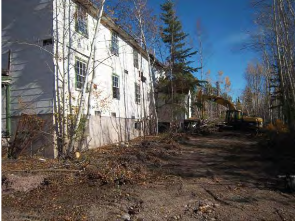
1161 – Demolition of apartment building #1.
