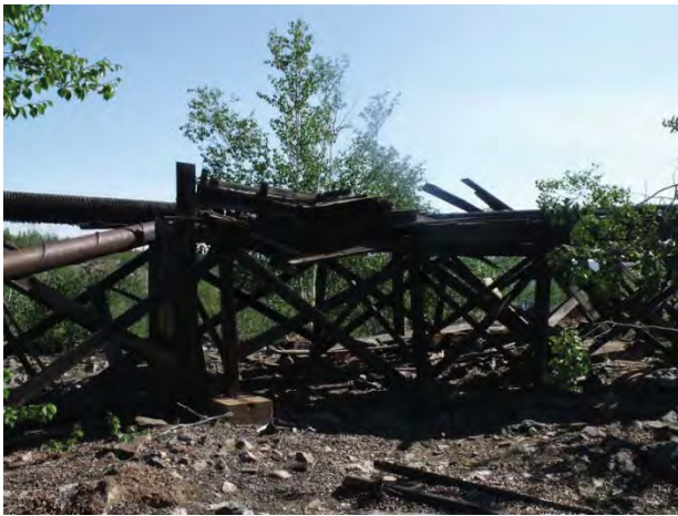
Photograph 115 ↑ Tailings and Utilidors-05
