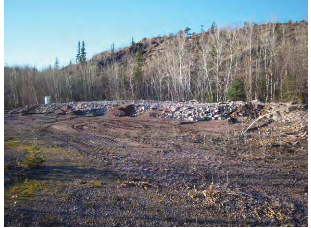
1235 – Debris covered with clean waste rock.
