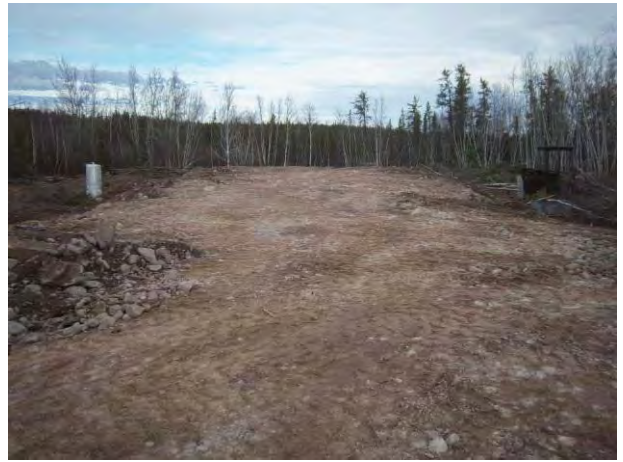
1266 – Debris covered with clean waste rock.
