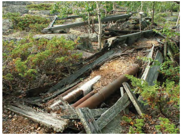
Photograph 116 ↑ Tailings and Utilidors-06
