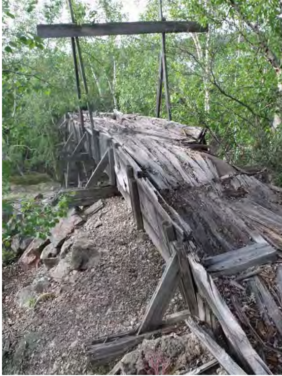
Photograph 117 ↑ Tailings and Utilidors-07
