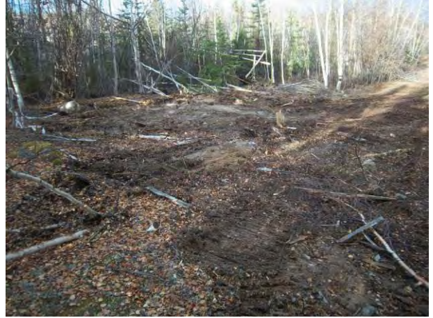
1295 – Removal of debris.
