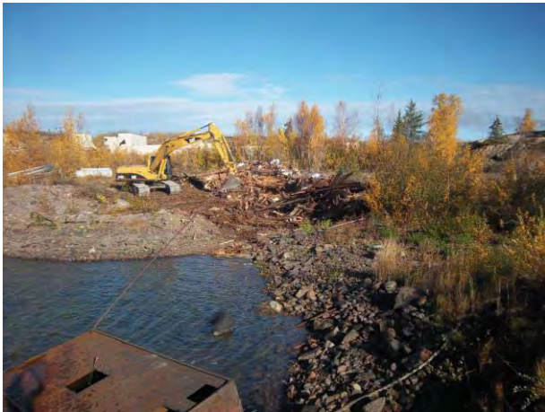
1104 – Demolition of the Barge.
