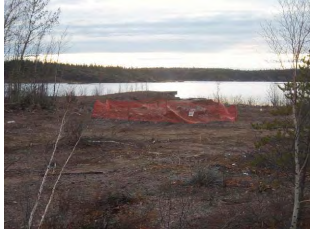
1344 – Debris covered with clean waste rock.
