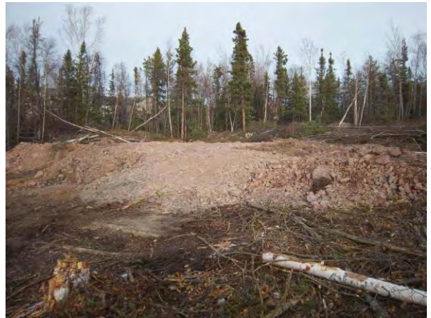
1254 – Debris covered with clean waste rock.
