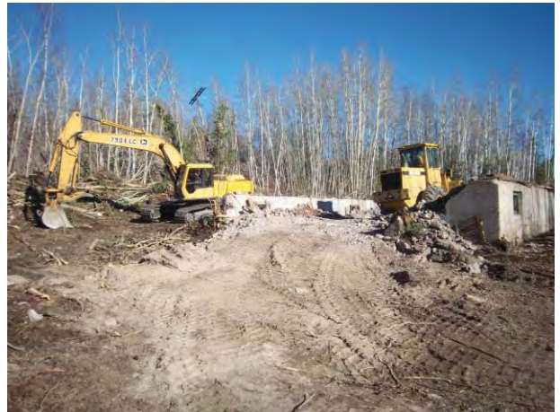
1248 – Debris covered with clean waste rock.
