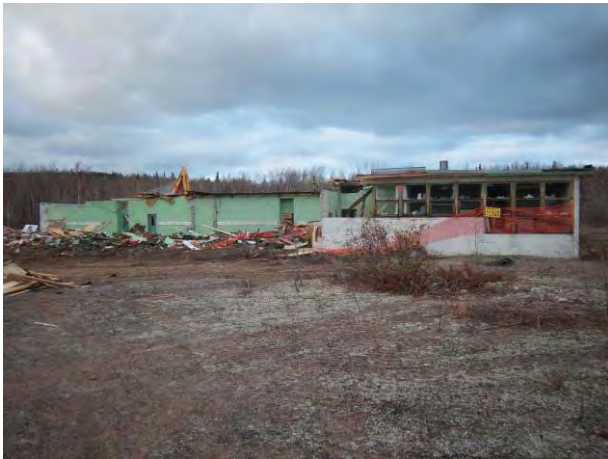
1376 – Demolition of the school.
