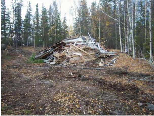
1182 – Demolition of west cabin from the marina.
