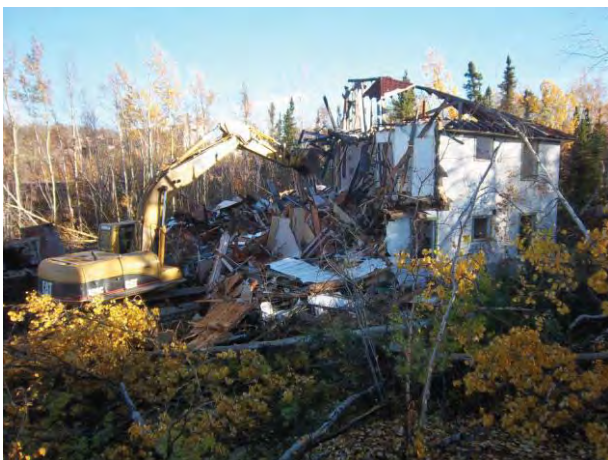
1156 – Demolition of the mine manager's residence.
