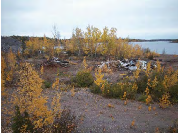
1099 – Demolition of the east cabins.
