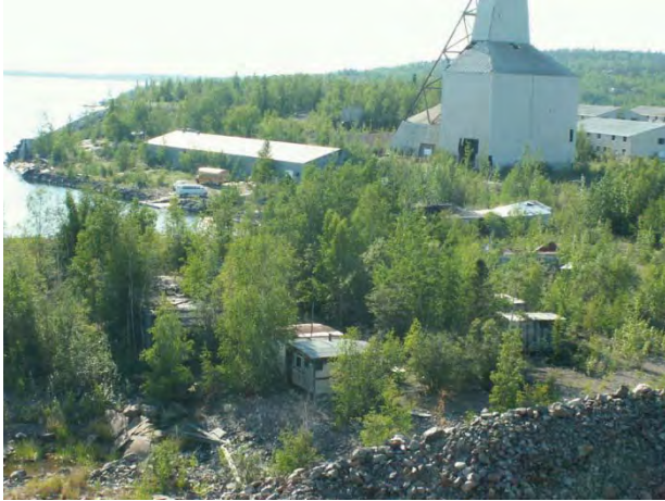
Photograph 29 ↑ Cabins East of Mine-01
