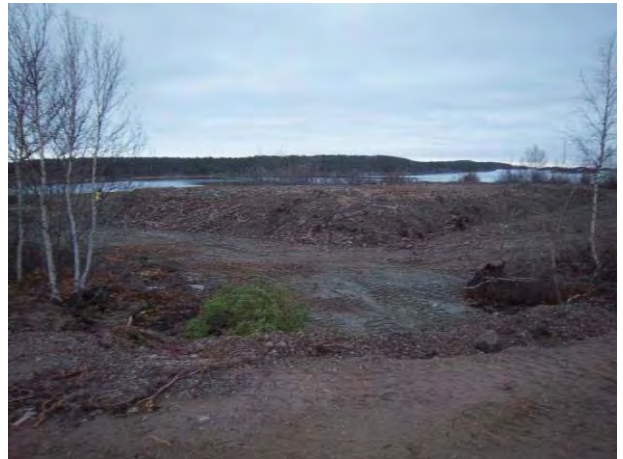
1394 – Debris covered with clean waste rock.
