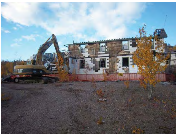
1108 – Demolition of bunk house #2
