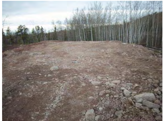
1290 – Debris covered with clean waste rock.
