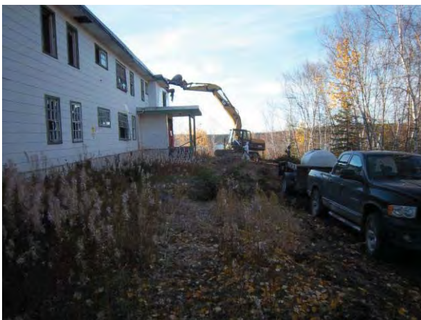
1181 – Demolition of apartment building #2.
