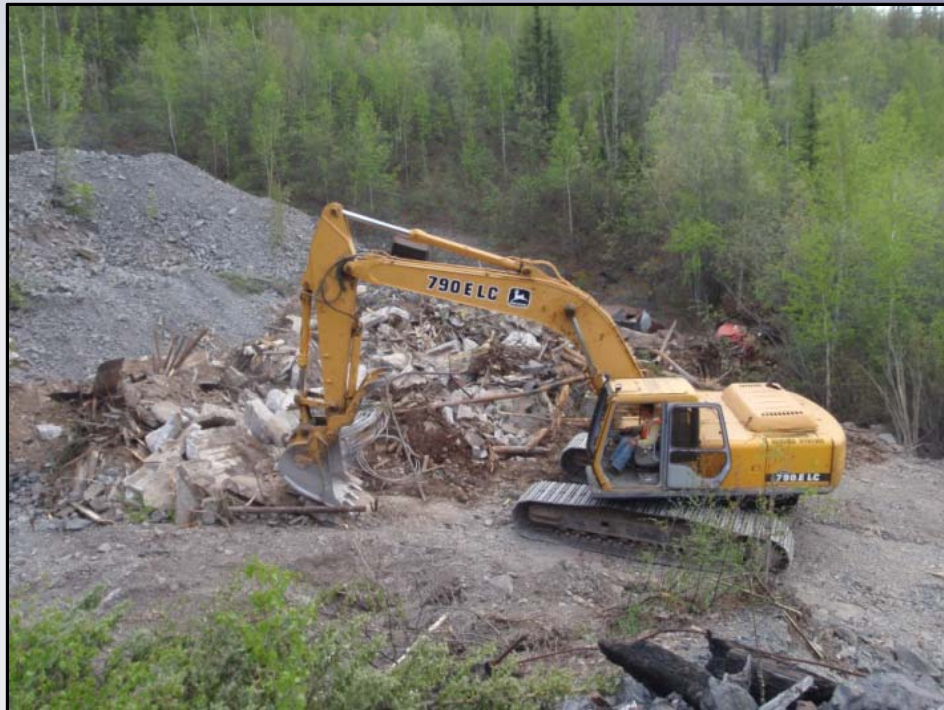
(left) debris disposal area
