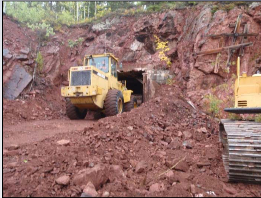
(left) Backfilling of the 1 st adit
