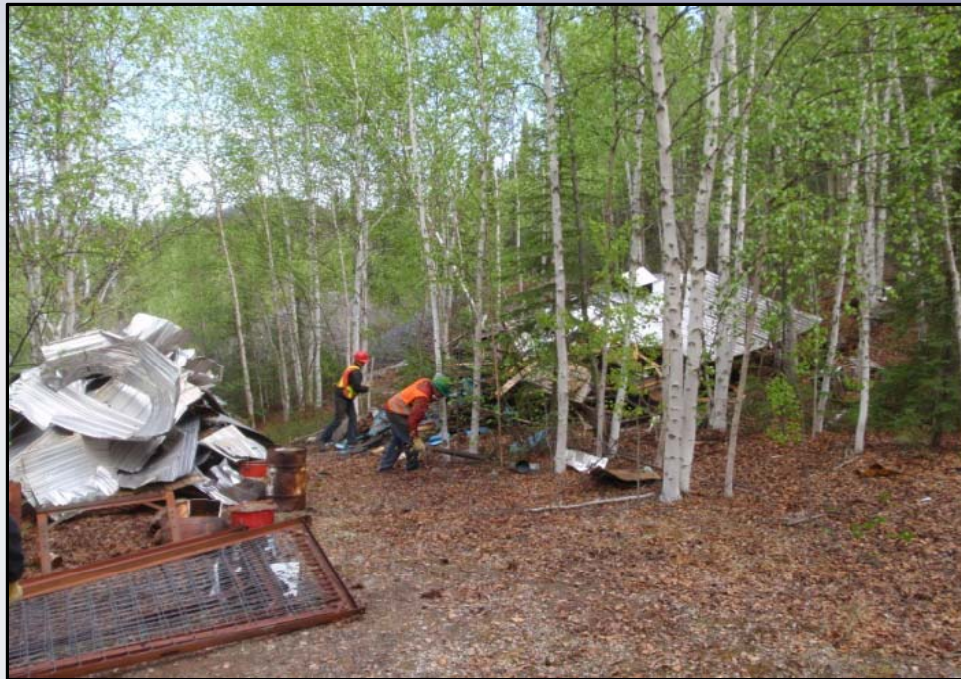
(left) dismantling of the tin shed
