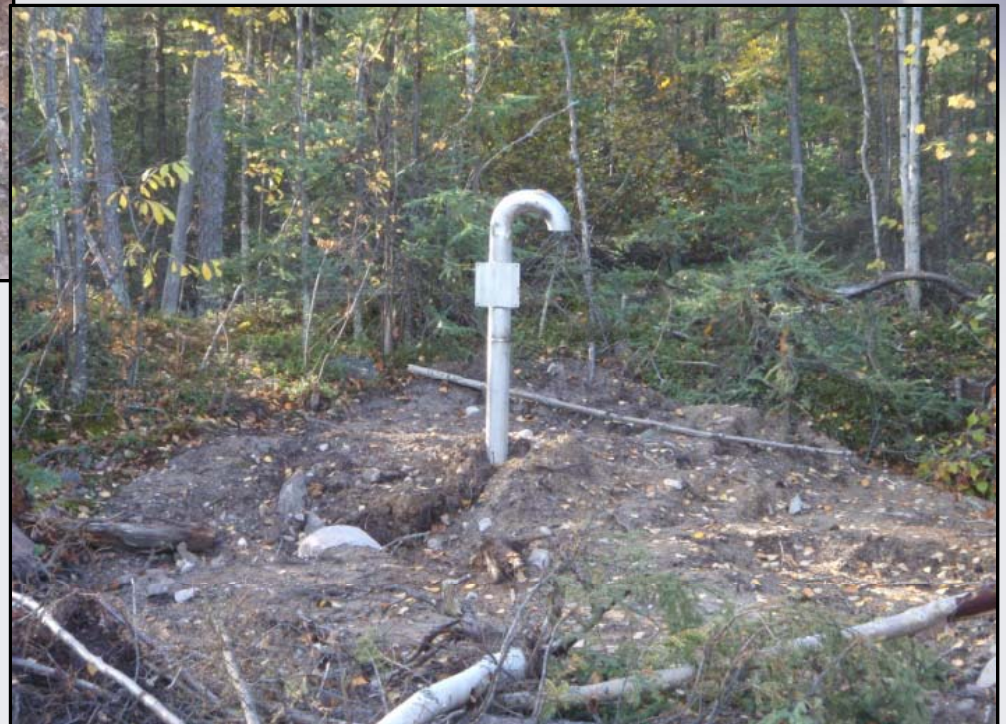
(right) Vented raise sealed with PUF.
