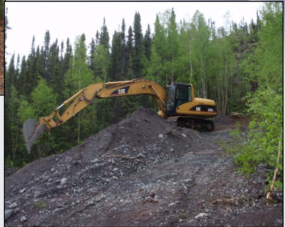
(right) contouring of the remaining waste rock
