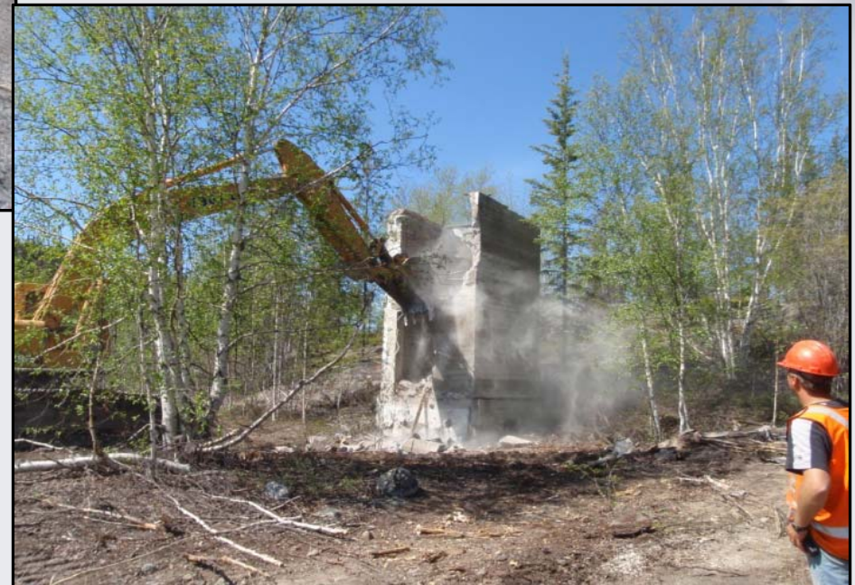
(right) demolition of 2 storey concrete structure
