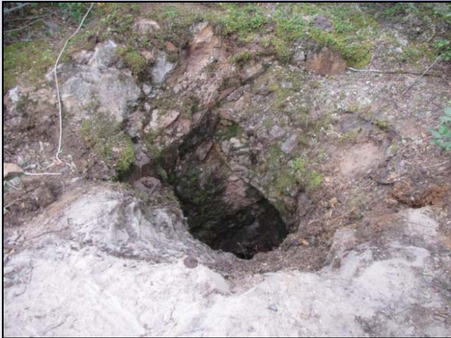
(left) Exposed opening of raise
