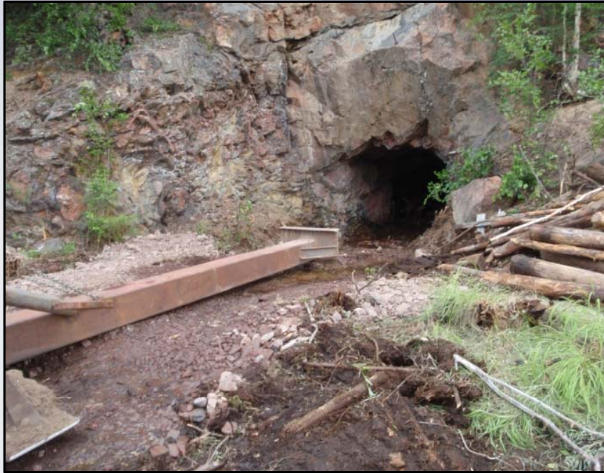
(left) adit opening prior to backfilling
