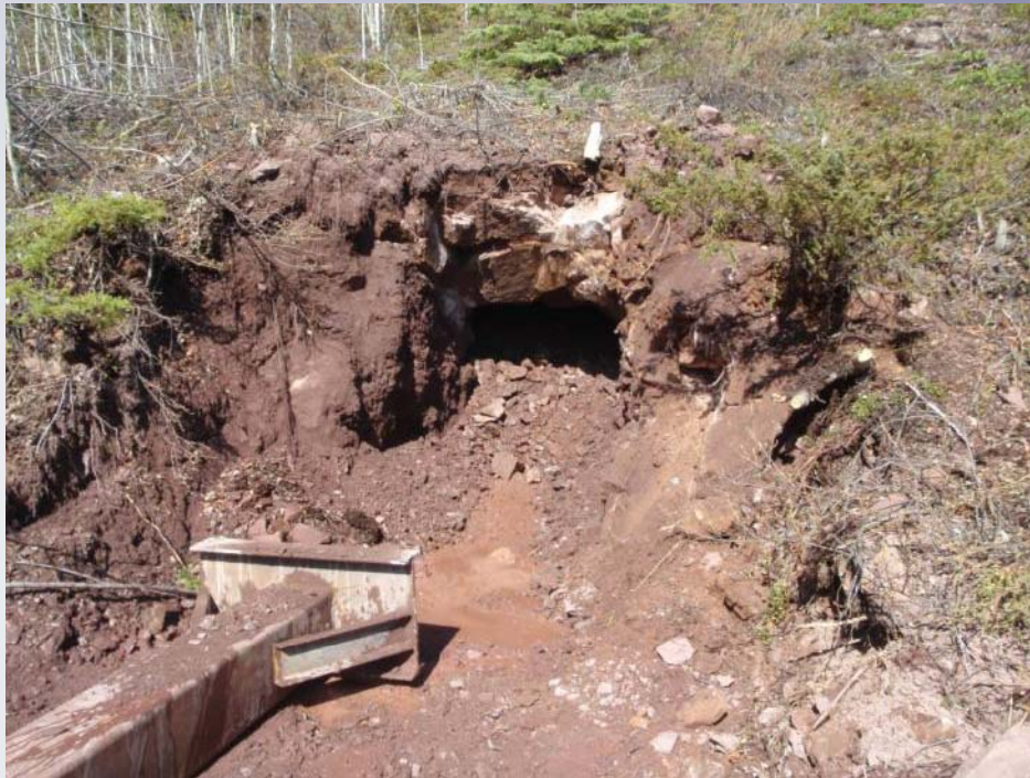
(left) backfilling of adit #1.
