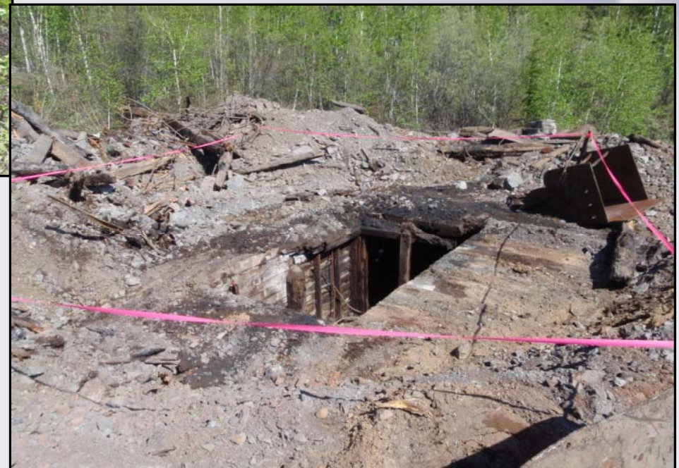
(right) debris removed from shaft opening.
