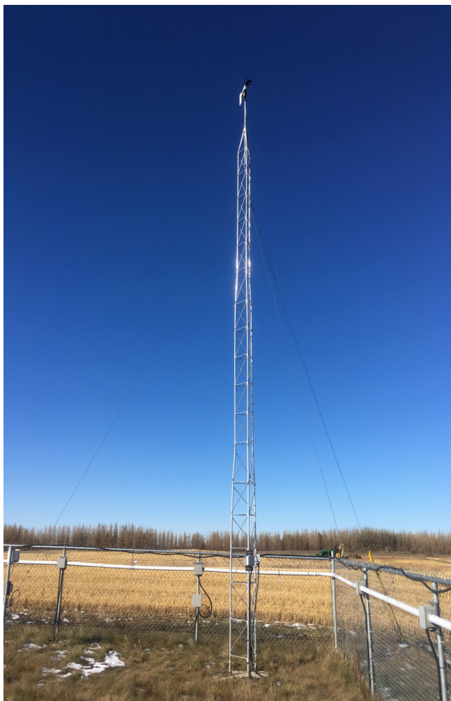
10 meter wind speed and direction tower October 2018 Photo: Development Engineering and Manufacturing
