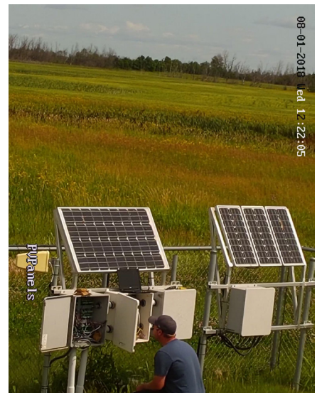
Site maintenance August 2018 Photo: Camera at site
