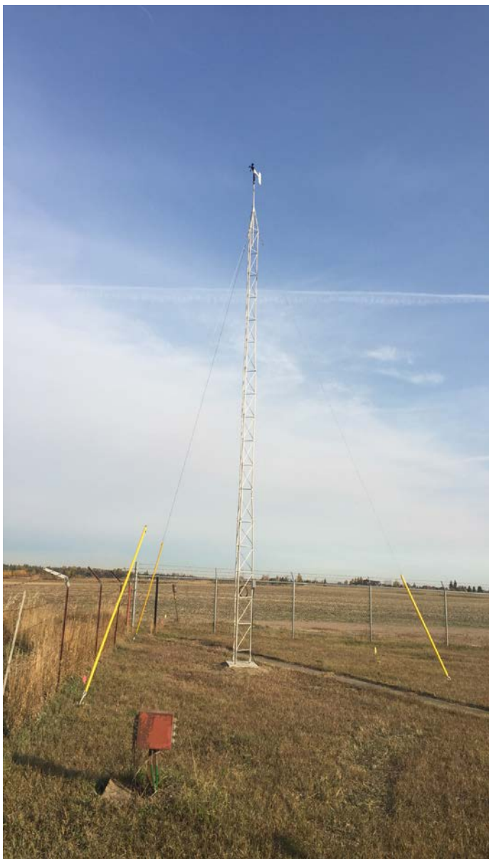
10 Metre Tower with Wind Speed and Direction 11 October 2017 photo: V. Wittrock
