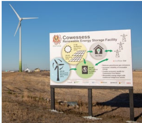
Cowessess Renewable Energy Storage Facility near Regina, SK
