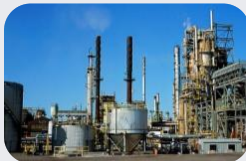
Point Sources – Oil refinery
