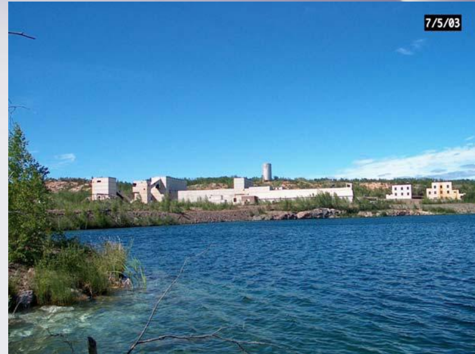
Crusher, Mill, Acid Plant
