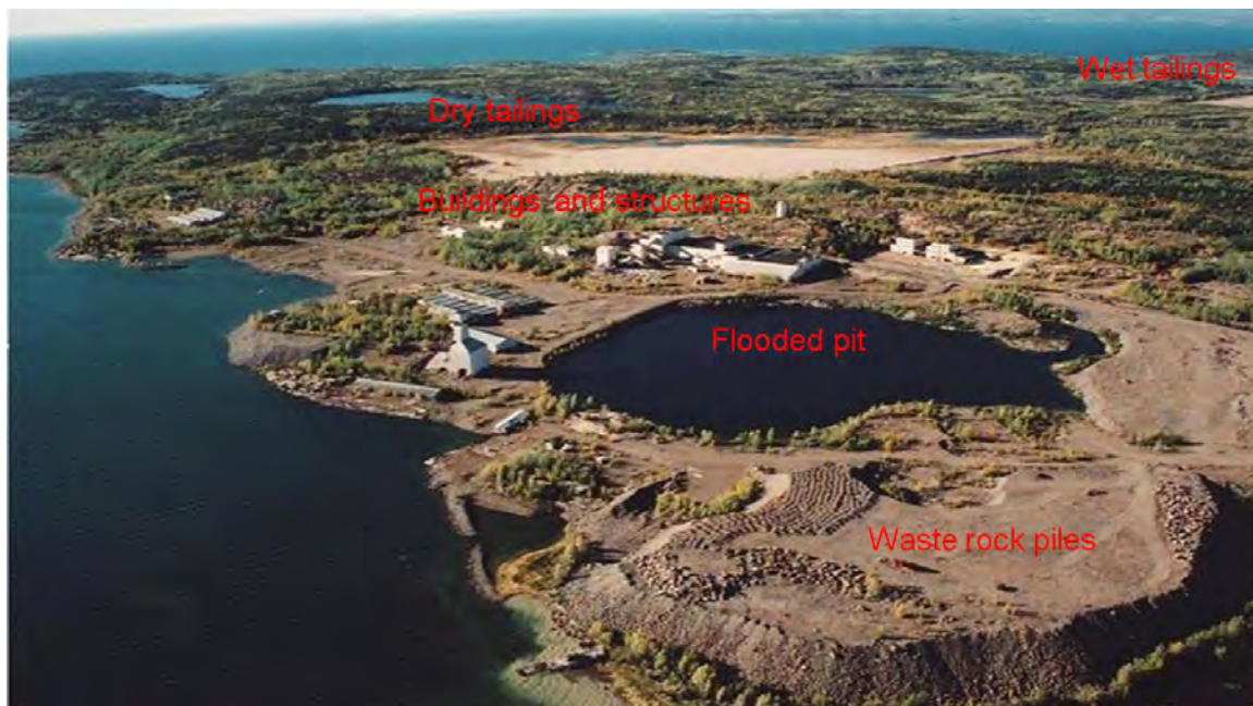
Figure 2. Gunnar mine site before demolition of buildings and structures (2009)
