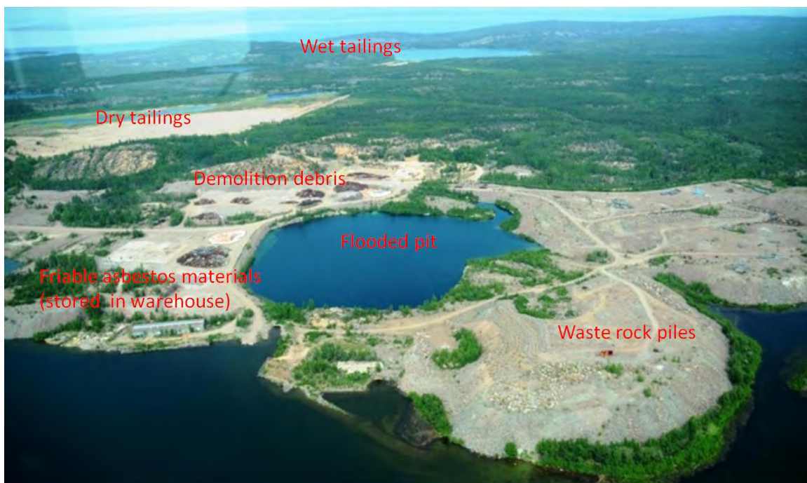
Figure 3. Gunnar mine site after the demolition activities (2013)
