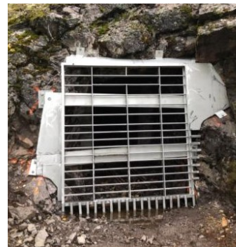
Stainless-steel grate installed at Meta Uranium Mines, Beaverlodge Lake, Umisk Island. The larger gap at the top of the grate is designed to allow bats in and out of the mine.
