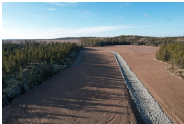
Completed Beaver Pond cover system and drainage channel
