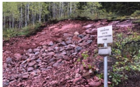
Adit 2 backfilled with rocks at Nesbitt Labine ABC Mine. The coarse material will allow drainage of mine water and prevent it from accumulating inside the mine.
