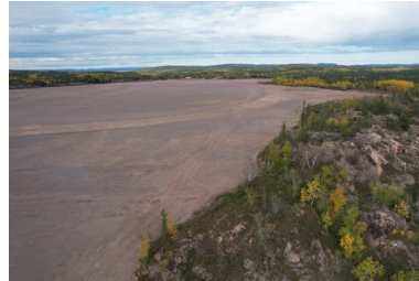
Completed Gunnar Main Tailings cover
