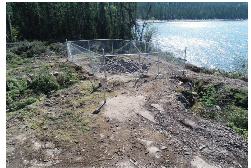
Pic 1: Backfilled shaft and remediation perimeter fence installed at Caba
