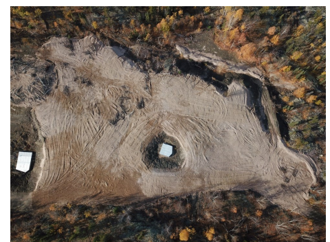
Pic 3: Sand cover at Lorado Mill
