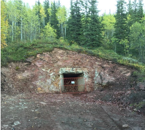
ABC Adit 2 Mine opening will be closed during the next field season
