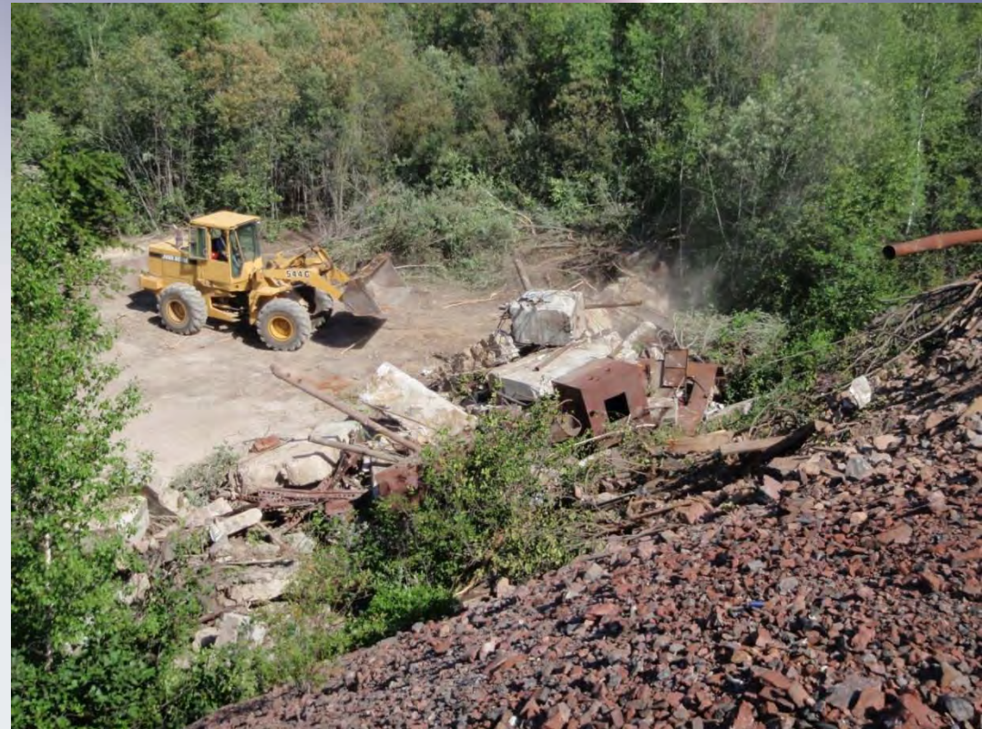
Concrete and steel being placed for burial with waste rock
