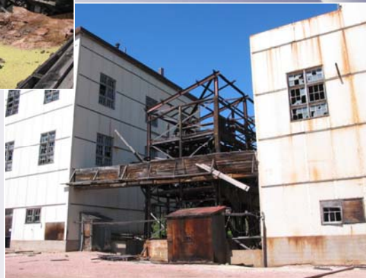
Acid Plant corroded and structurally unsound
